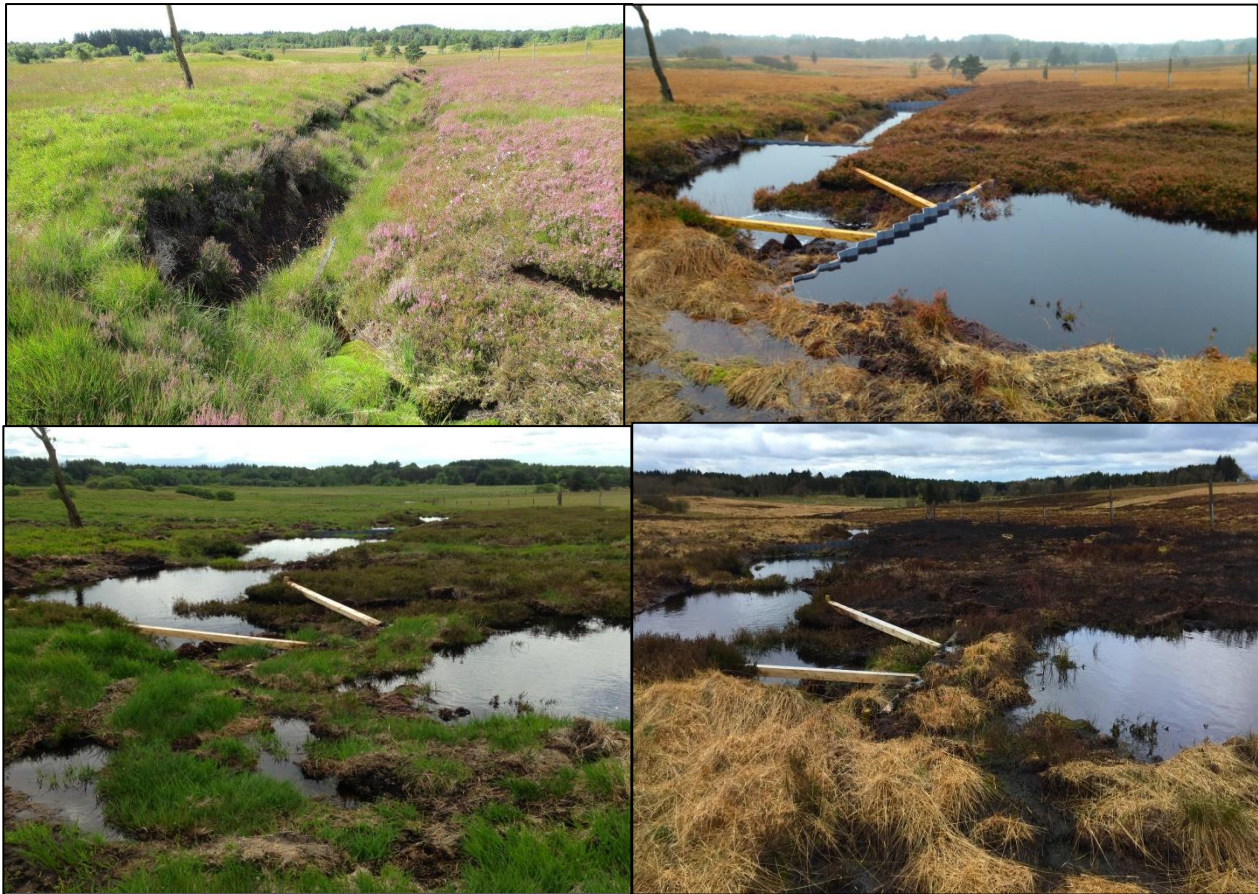
Figure 4. Large blocked ditch in Compartment 2 at Fannyside Muir helped to constrain spread of fire in April 2017
