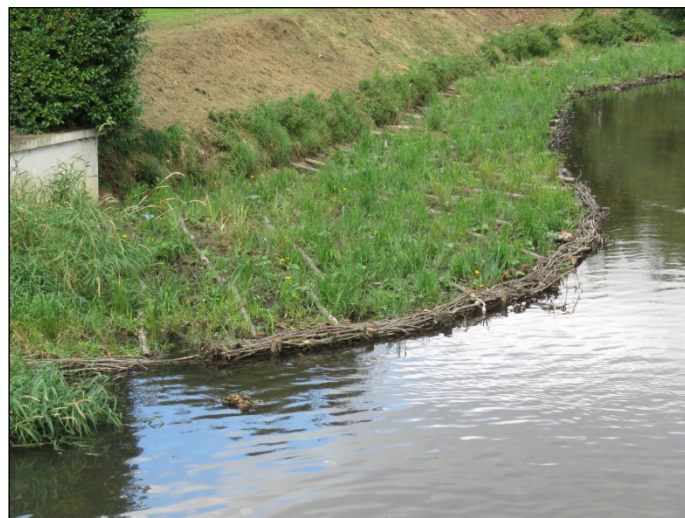
Close up of planted soft berm enclosure showing edging of faggots and top of pre-planted coir rolls.
