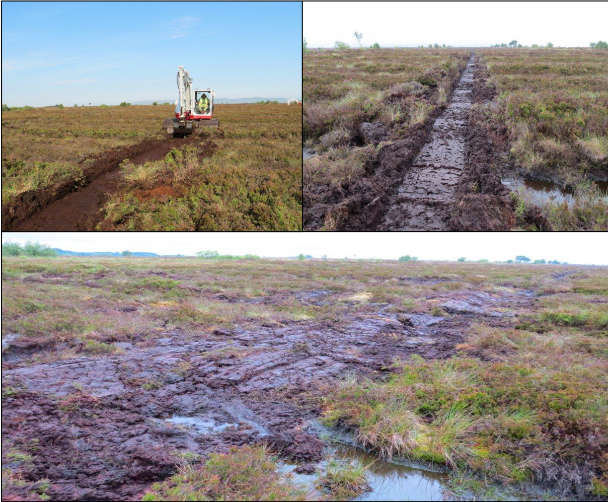
Figure 1. Installation of trench bund in Compartment 13a.
