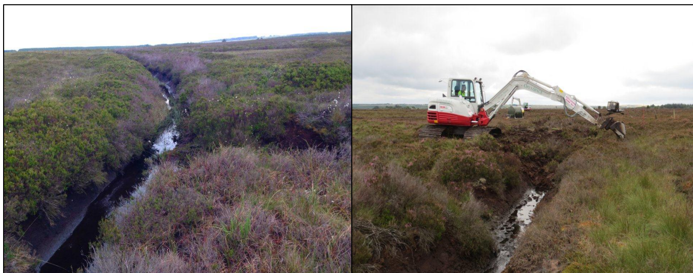
Figure 5. Reprofiling steep-sided boundary ditch.
